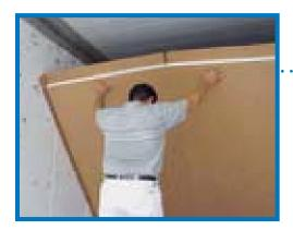
Gradually lift the bulkhead into place. The "spacer pallets" will prevent the bulkhead from sliding.
