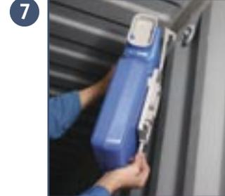
Using a stepladder and holding the bottom of the hook bar, lift the unit up all the way up to the ceiling and place the hook on the loop in the container wall.
